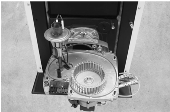
Abb. 36: Brenner in Serviceposition
