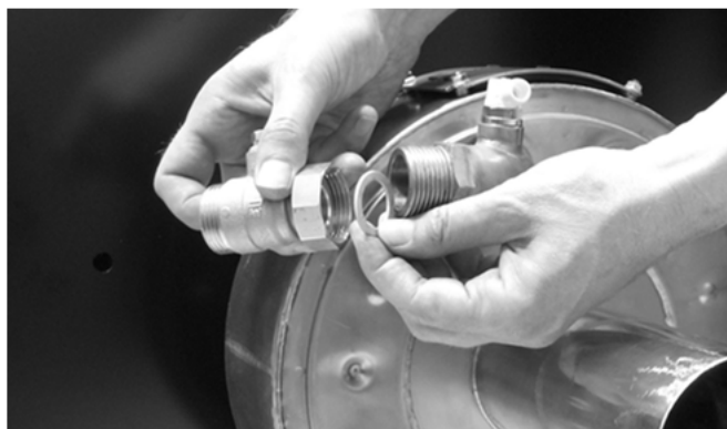
Abb. 28: Montage Kugelhahn 1"
